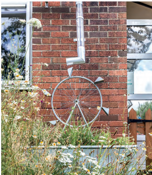
ABOVE: The water wheel, fed by an overflow downpipe, adds an exciting visual feature to a rain planter within an Action for the River Kennet project designed by Wendy Allen. BELOW: An eye-catching arrangement of downpipes draws attention to a series of filtration rain planters which Wendy designed to slow the flow of rainwater off the buildings of Preshute School.
