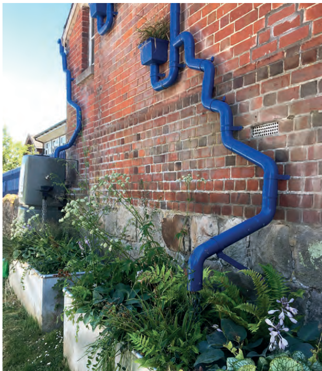
ABOVE: The water wheel, fed by an overflow downpipe, adds an exciting visual feature to a rain planter within an Action for the River Kennet project designed by Wendy Allen. BELOW: An eye-catching arrangement of downpipes draws attention to a series of filtration rain planters which Wendy designed to slow the flow of rainwater off the buildings of Preshute School.
