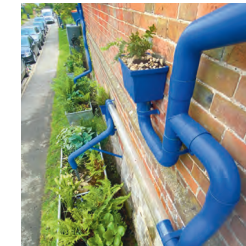
Shalbourne School rain garden (top), and rain planters and downpipes for Preshute School, both by Wendy Allen Designs for Action for the River Kennet.
